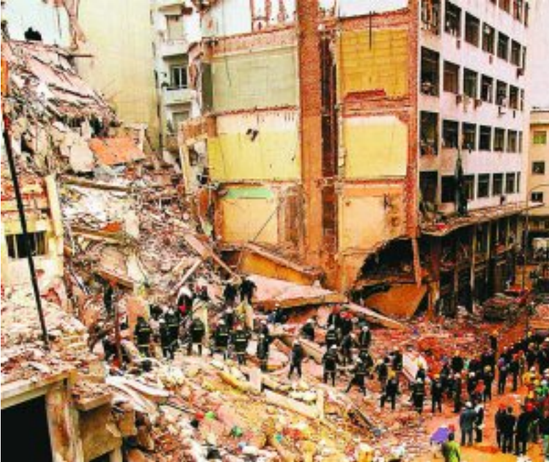
Figure 4: Rubble of the AMIA building after the July 1994 Car Bombing
