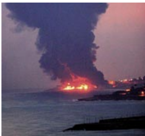
Clouds of smoke from Jiyeh power station in Lebanon
