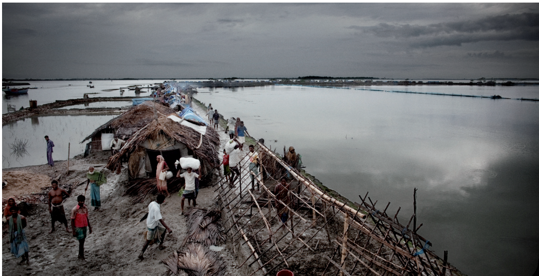
Flood defences on the island of Padma Pakur, Bangladesh. Between the village and the water, trees have been planted to prevent erosion and act as a shield against the wind.
