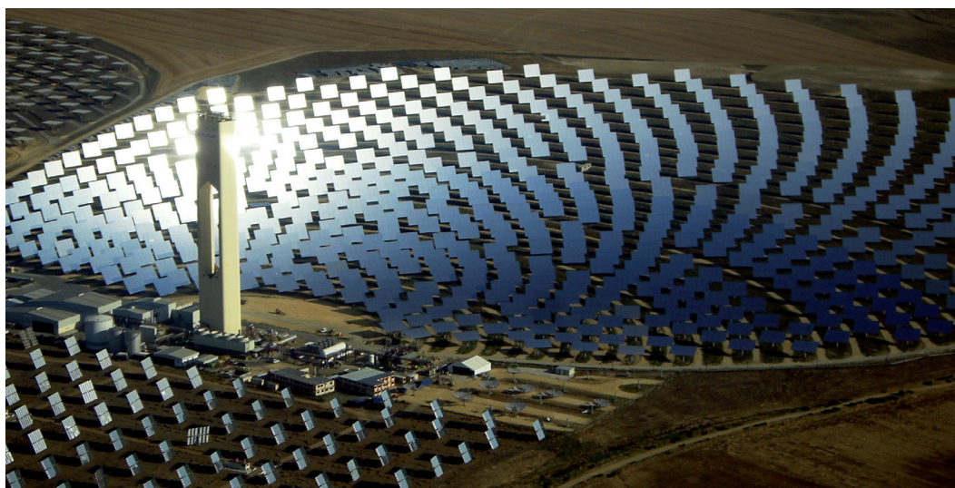
In Spain, new solar panel plant PS20 is under construction next to plant PS10. At a height of 115 metres, PS10 is powered by 624 mirrored heliostats. At 165 metres, PS20 is powered by 1 255 of them. PS20 has been designed to produce twice the energy of its smaller, 11 MW neighbour. Although not the world's first 'power towers', these are the first such plants conceived on such a scale.
