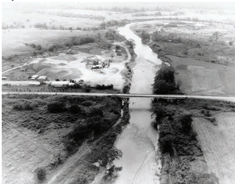
Pacora River Bridge.
