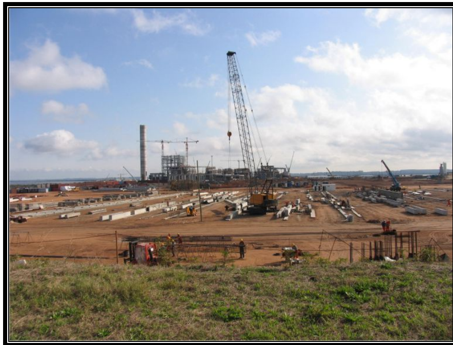
Figure E5.1-3: Botnia Mill Site Under Construction, Looking Toward the River
