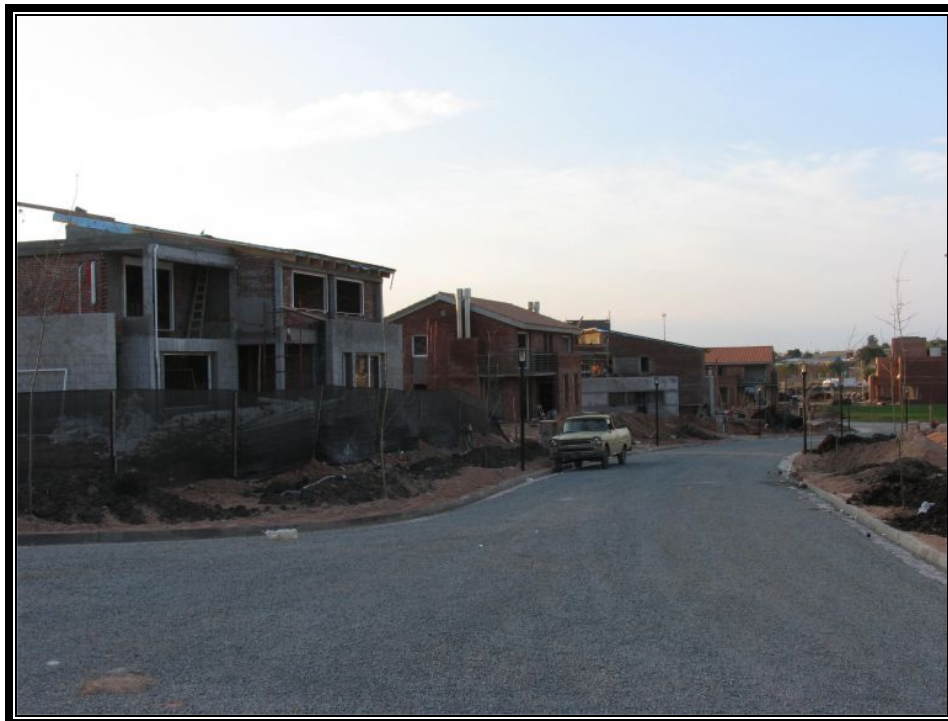
Figure E5.1-7: Botnia Housing Project in Fray Bentos
