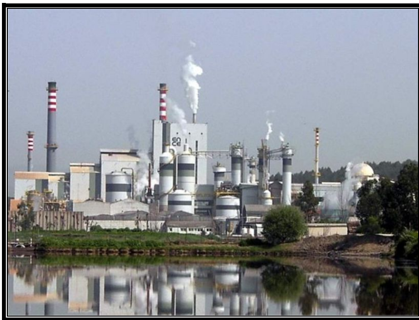
Figure E5.1-16: ENCE Mill Operating in Spain
