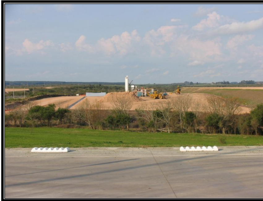
Figure E5.1-4: ENCE Mill Site, Preparation for Construction
