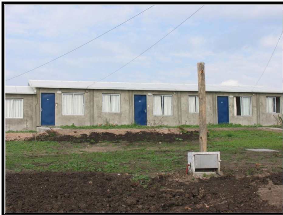
Figure E5.1-9: Finished Employee Housing, Fray Bentos. Designed for single immigrant construction workers.
