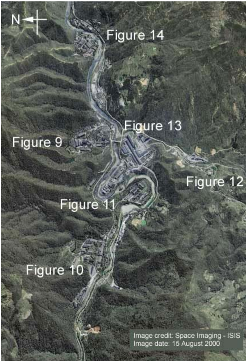
Figure 8 -- Overview of facilities at the nuclear site at Guangyuan.
